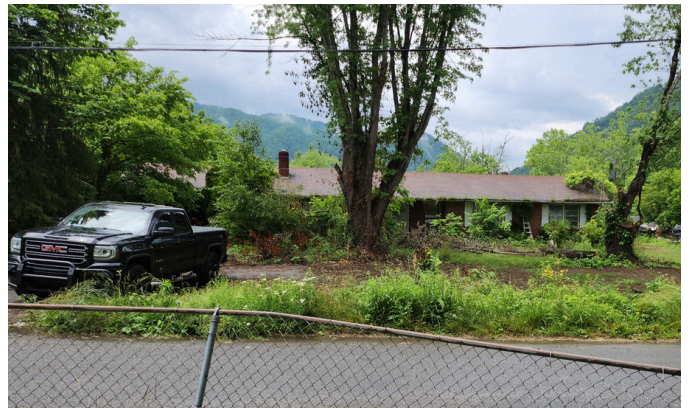
The abandoned house across the street
